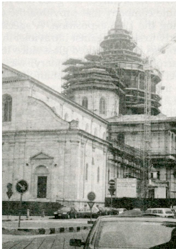
Restoration on the roof began last January. Photo by D.C.
